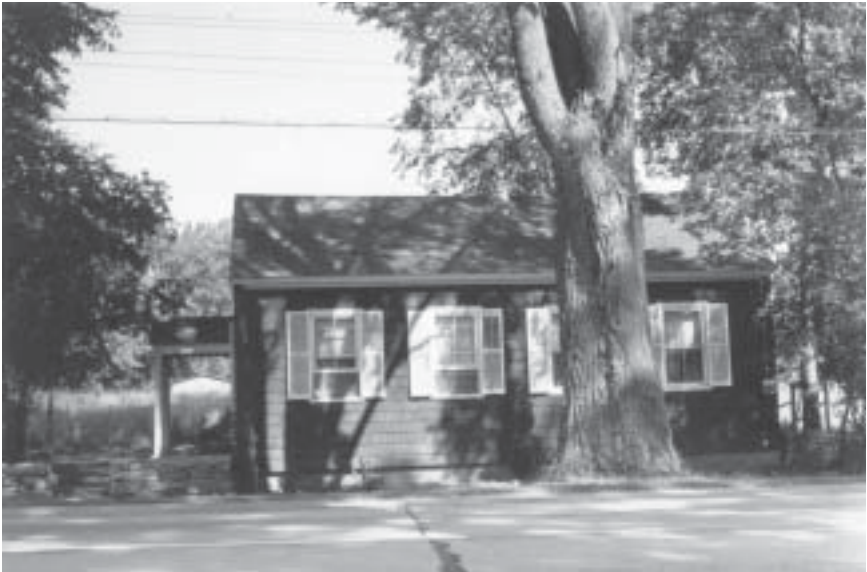
School House on East Street
