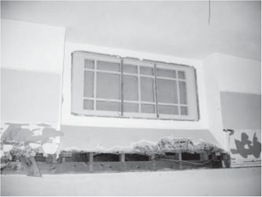
Hidden windows from classroom into hallway
