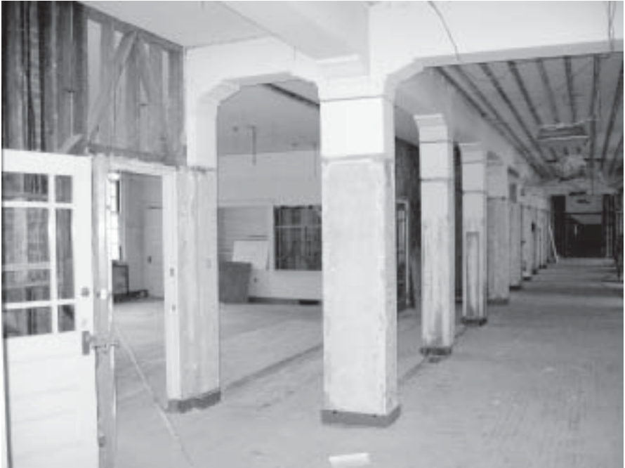
Original columns with a view of the future Selectmen's Office
