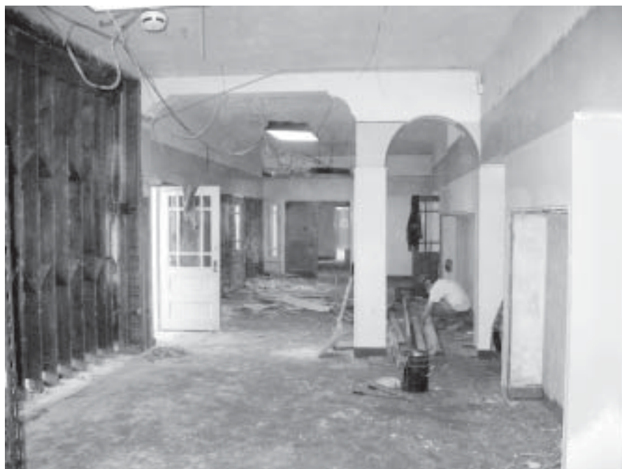
Arch detail on second floor.
