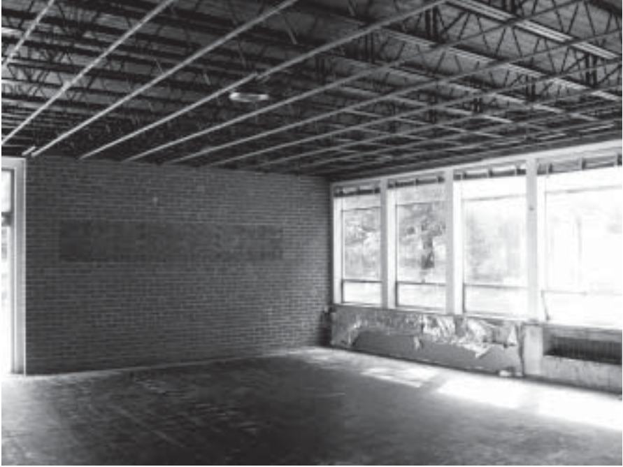
First floor of the future Police Station
