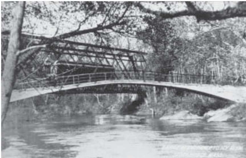
Goodrich Memorial Bridge - Property of Laurel Hill
