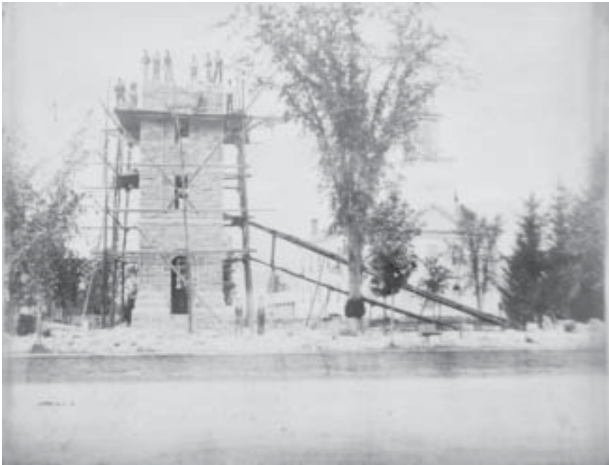
Children's Chime Tower - Work in progress.
